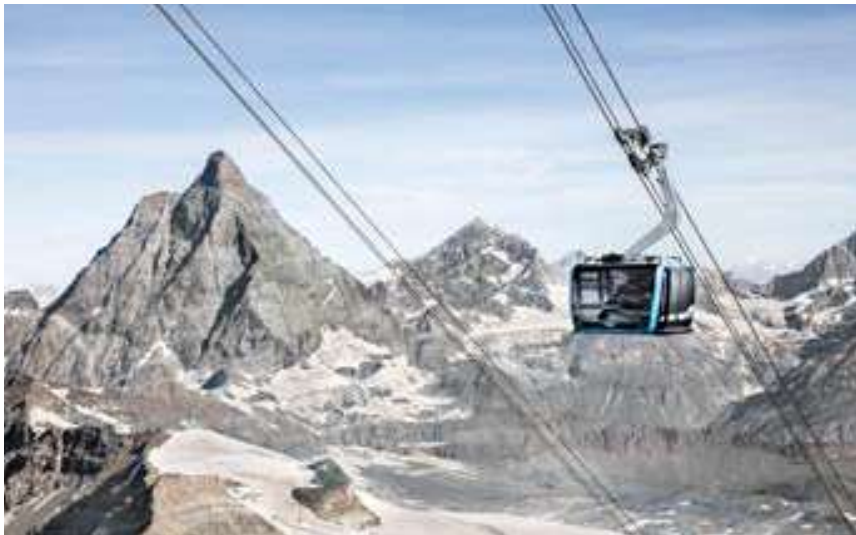
Matterhorn with 3S cableway, Zermatt, Valais
