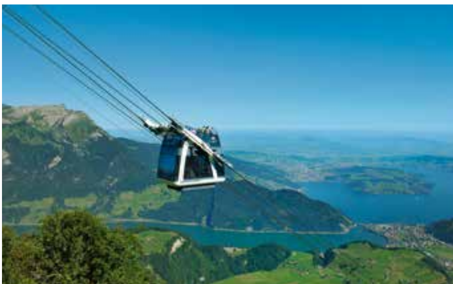
CabriO cableway, Stanserhorn, Lake Lucerne
