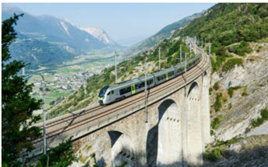
BLS RegioExpress Lötschberger on the Luogelkin Viaduct at Hochtenn, Valais
